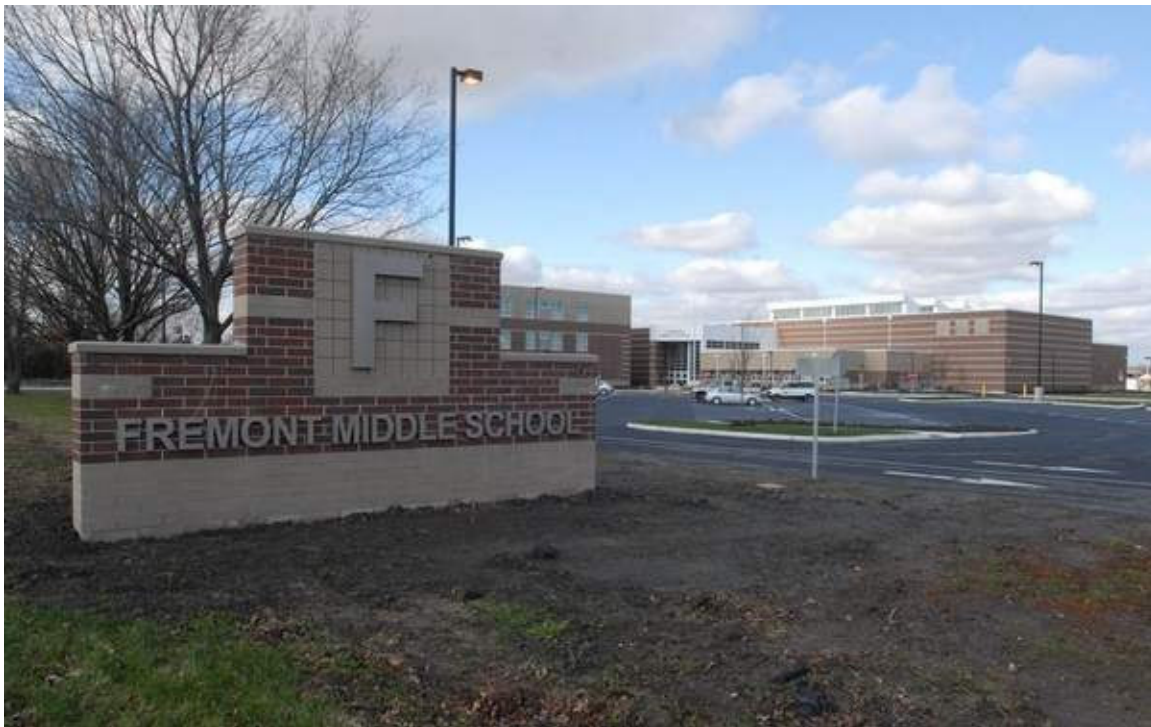
The new Fremont Middle School, which encompasses 126,000 square feet and cost $25 million to build, will welcome its first students Jan. 19.
