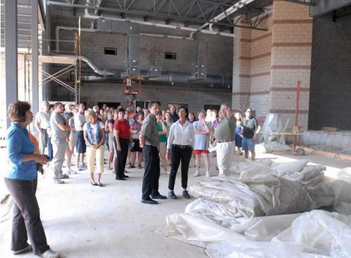
Staff of the Fremont City Schools tour the construction site of the new Fremont Middle School on Tuesday. / Jonathon Bird/News-Messenger
