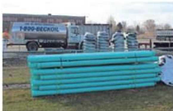
Early site work and stacks of supplies were evident at Croghan Elementary School.
